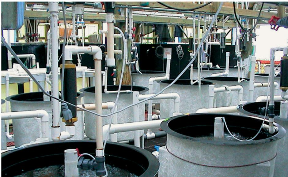
Changes to reduce bacteria levels in the research hatchery included improved system design, better management and the optimization of pipe sizes and reduction of by-passes and other regions where bacteria might accumulate.
