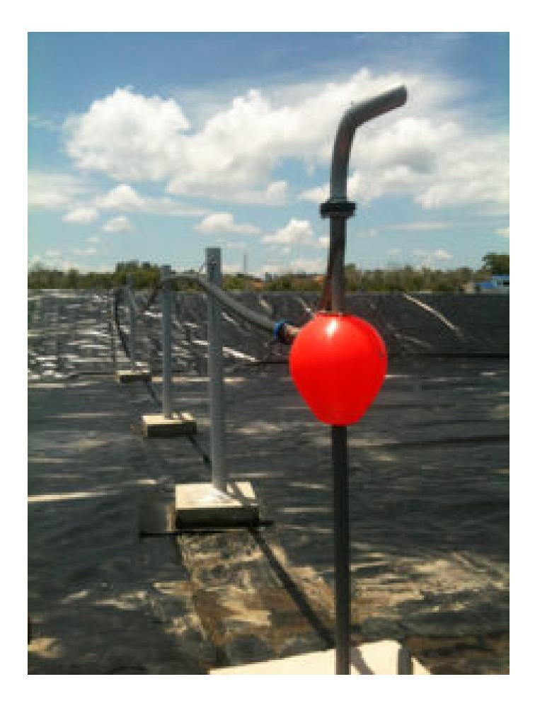
A central, computer-controlled system distributes feed to individual ponds for distribution through rotating spreaders.
