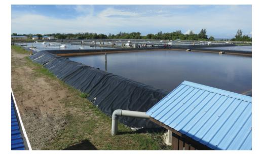
The Brunei operation uses three-stage treatment ponds that settle out solids and detoxify wastewater before recirculating it back into the production ponds.
