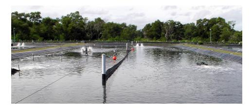
In addition to ponds operated with counter-rotating aeration "cells," a "carousel" system incorporated a central divider and
