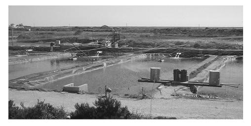
The experimental seaweed biofilter system operated at an intensive sea bream farm in southern Portugal, where flow-through fish ponds continuously supplied 12 seaweed biofilter tanks.
