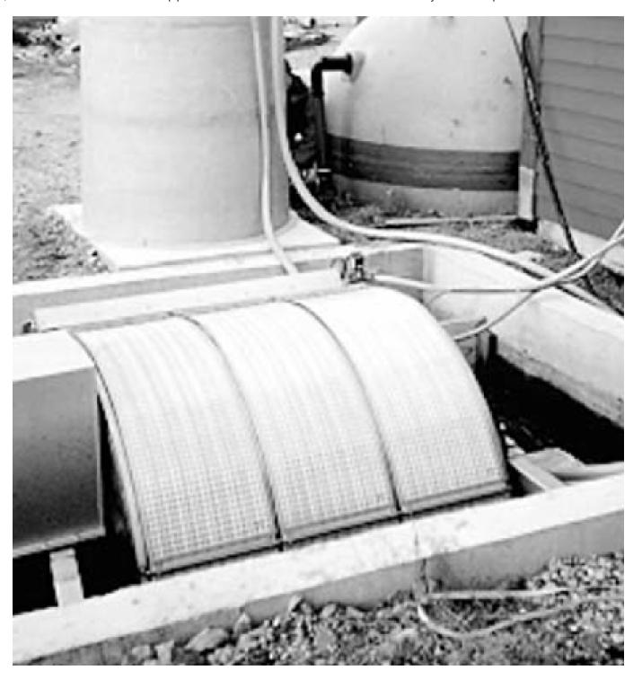
The effluent treatment system described at a hatchery in County Rogaland (Bokn Settefisk). The main units are a drum sieve, a thickening tank (tubular) and a unit for sludge stabilization.
