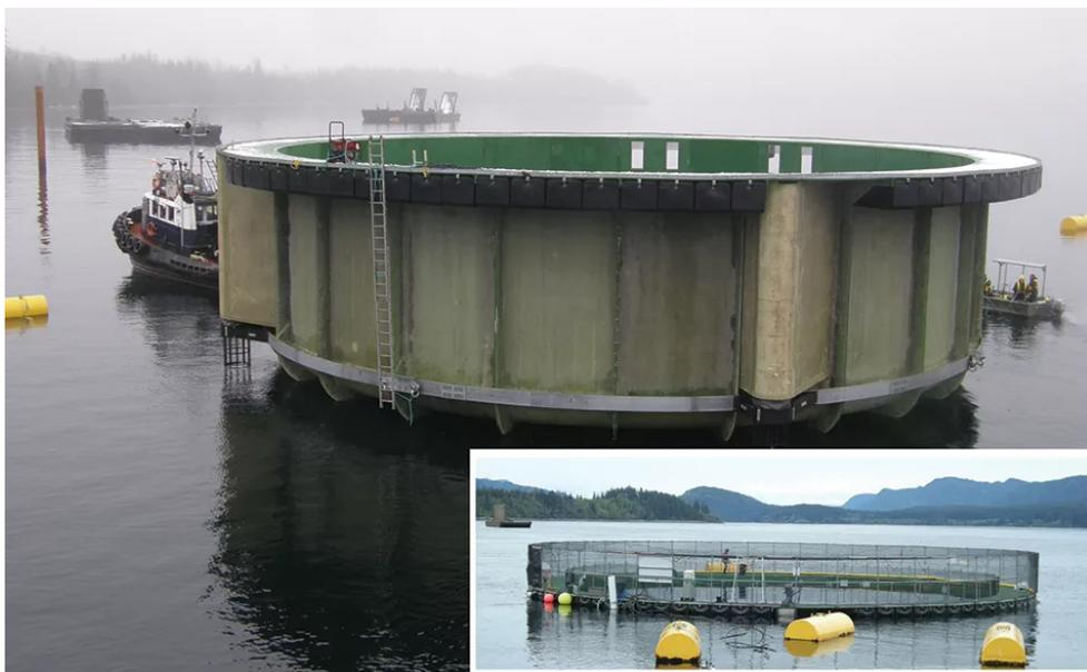
Solid-wall tanks are towed into position and “sunk” to a defined level.
