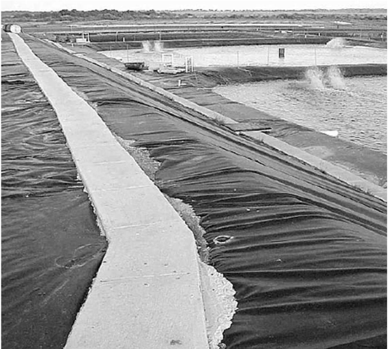
Fig. 2: View from elevated nursery ponds to grow-out ponds below. White nursery-to-growout transfer pipes protrude from the levee.
