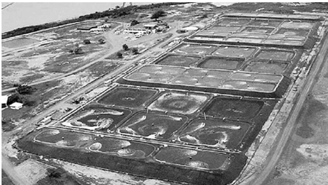
Fig. 1: Thirty-six intensive lined ponds were constructed adjacent to existing extensive earthen ponds.
