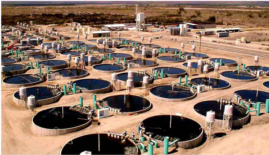
Kent SeaTech Corp. operates a successful high-density tank culture system that uses geothermal groundwater and biofilter systems to produce market-size bass. Photo by Jim Carlberg.
