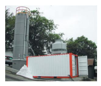
New self-contained mobile systems feature "containerized" ice slurry generation, pumping and controls.
