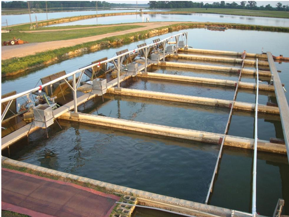
Paddlewheels on the upstream side of the raceways allowed frequent water exchange within the closed pond system.
