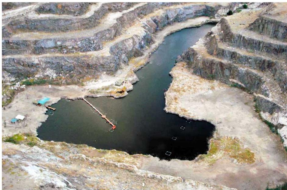
The lake formed when a tin mine eventually dug into an underground aquifer.
