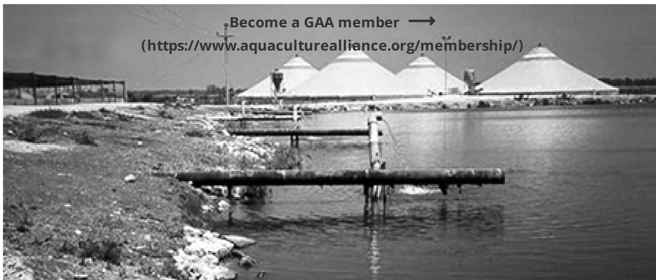
Intensive greenhouse-covered activated suspension ponds (background) connected to a water reservoir (foreground) in a closed cycle. Location: Negev Desert, Israel.
