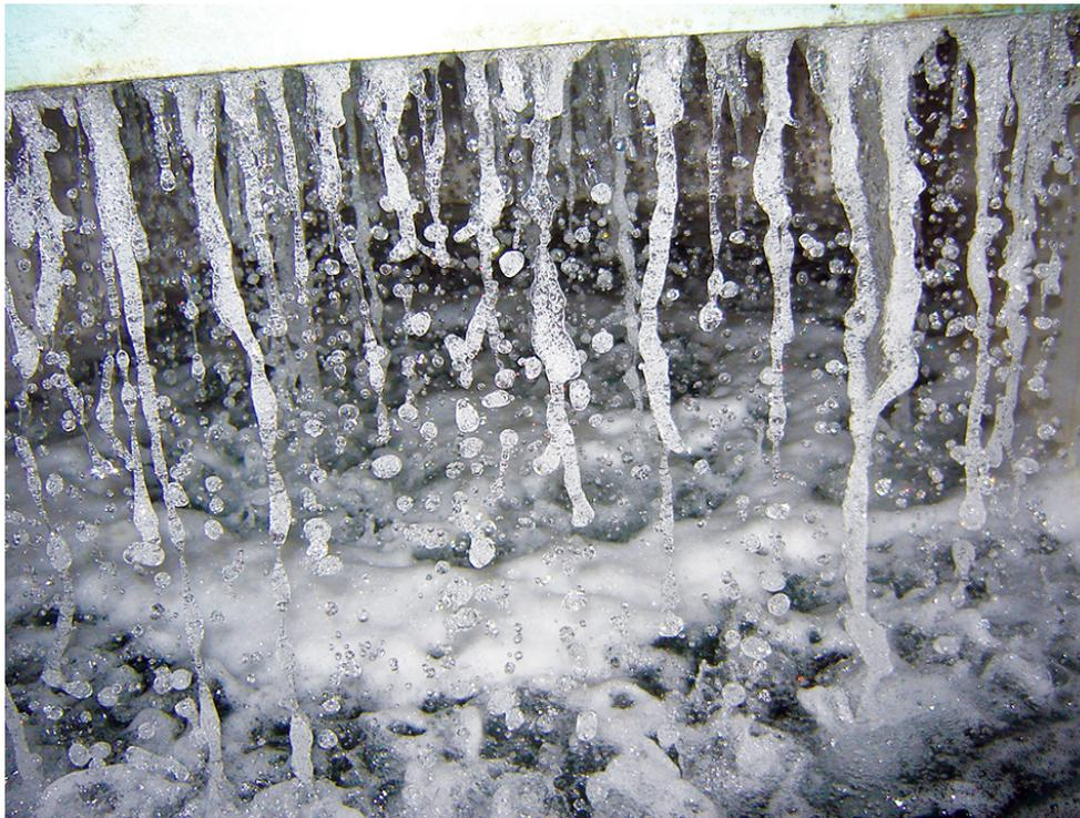
The discharge of a simple degasser helps partial pressures equalize by increasing air-water interface area.
