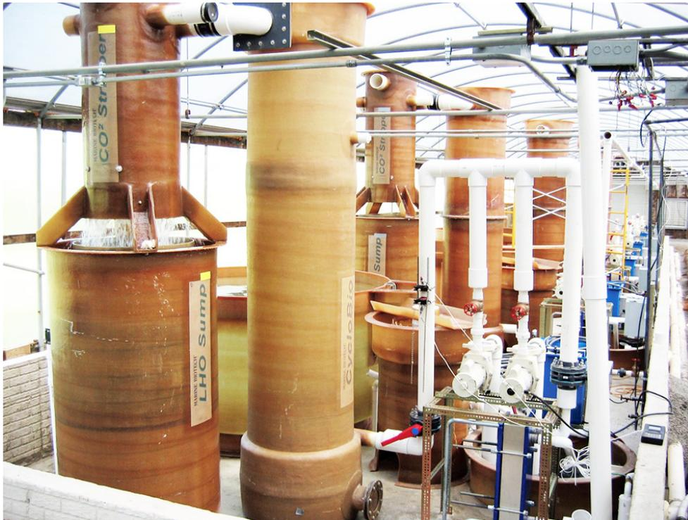
Compact yet powerful fluidized sand biofilters utilize sand particles to provide area for nitrifying bacteria to live and consume potentially toxic ammonia and nitrite-nitrogen. This Cyclo-BioFilter system uses tangential flow to reduce the energy required to expand the sand bed. Courtesy photo.
