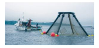
The low-tech OCAT system has proven viable as a fish containment structure for surface and submerged operations.
