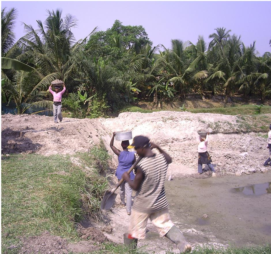
Most ponds in Ghana are manually constructed in a labor-intensive process that results in small, shallow ponds.
