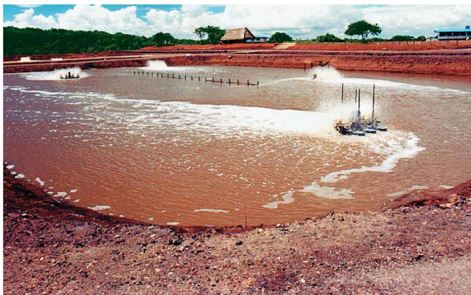
Aerators generate strong water movement in production ponds at the test facility.
